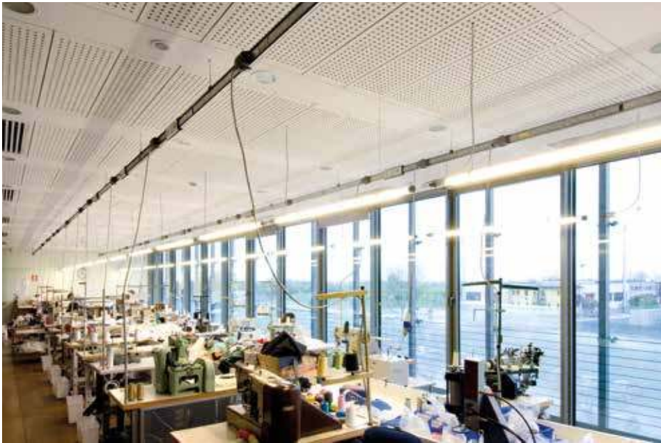
Example of lighting and small power distribution
